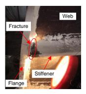
(b) Stiffener-to-flange weld fracture
